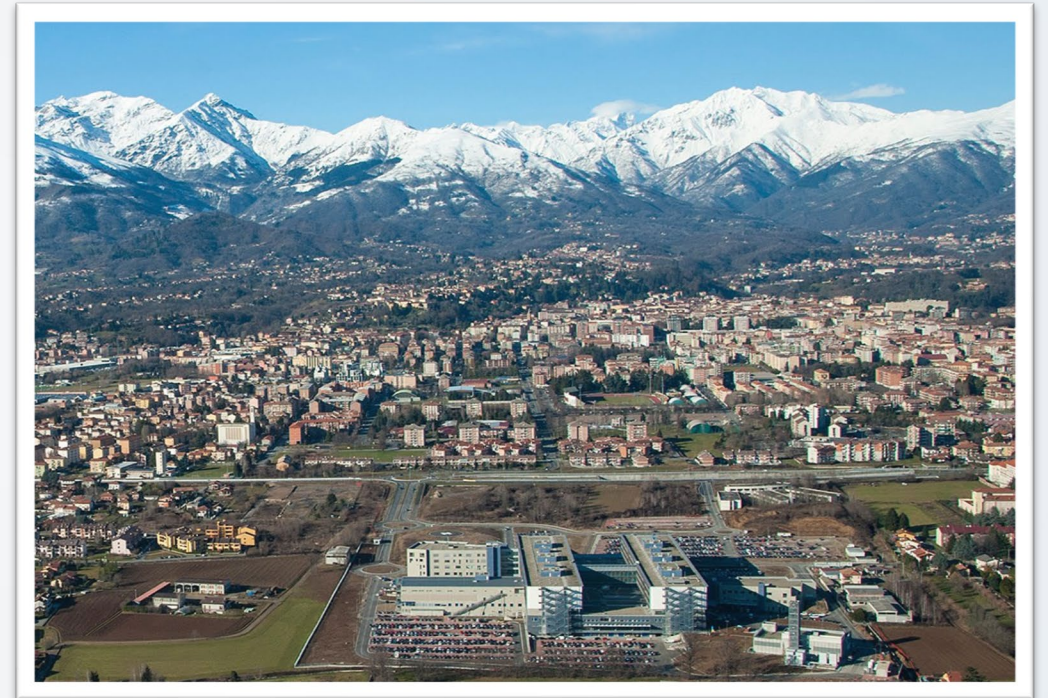
The New Biella General Hospital
